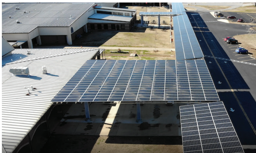
GOT IT COVERED —About 700 solar panels cover the arrival and departure canopy at Batesville School District's junior and senior high school.
